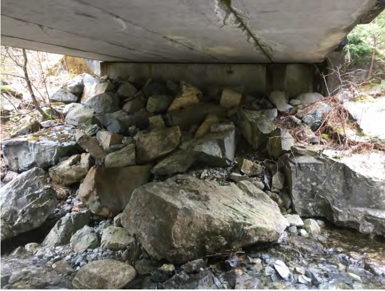
Right Bank Abutment when facing downstream
