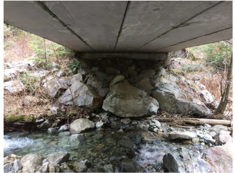
Left Bank Abutment when facing downstream
